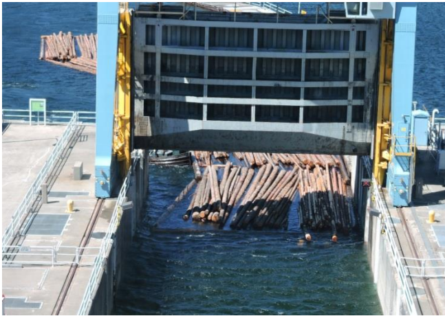
Raft entering the lock.
