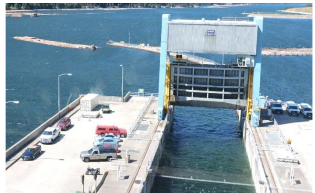
Raft approaching the lock with gate open and water at Arrow Lakes level.
